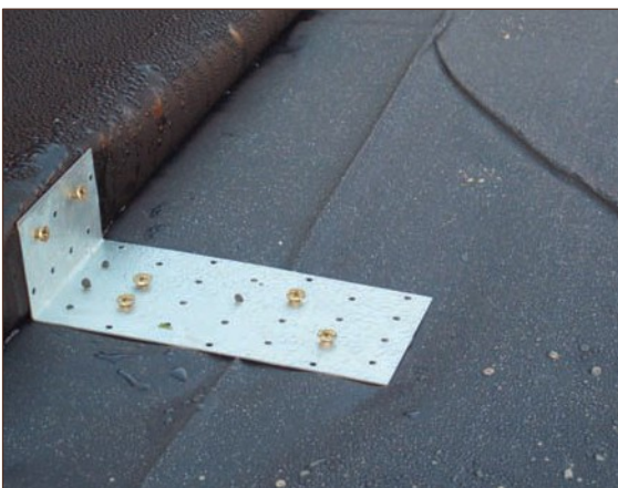
Figure A4.47 Follow-on works purposefully penetrating gas membrane (courtesy Card Geotechnics Limited)
