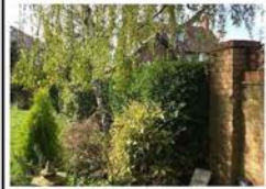
Figure 1. View of rear brick boundary wall towards the rear of garage
