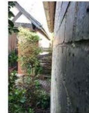
Figure 5. View from side of garage at No. 54 towards the rear
