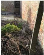
Figure 2. View of concrete post that delineates boundary towards the rear of garage
