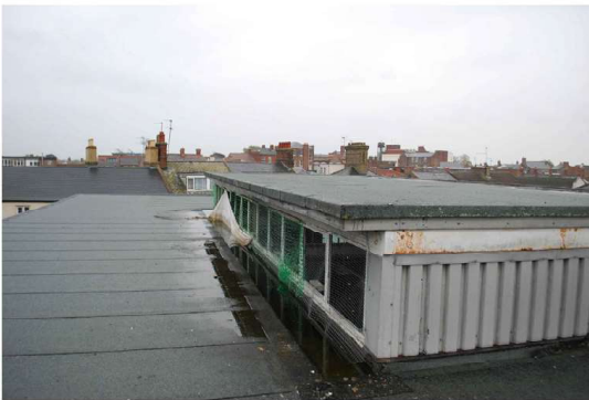
Above: Photograph at Roof Level, showing the Higher Section
