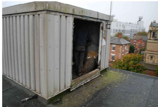
Above: Photograph at Roof Level, showing the Cat Ladder Tower
