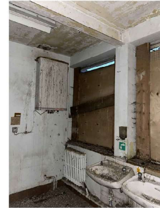
Above: Existing Mezzanine Level Area's
