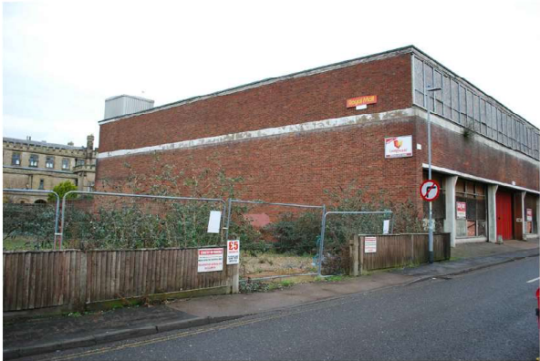
Above: View from Spring Gardens, overlooking the rear park
