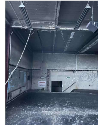
Above: Existing First Floor, Open Plan layout with exposed structure
