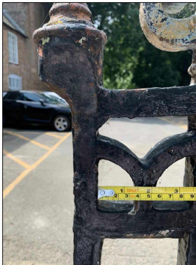
Head detail over meeting stile - North gate Note: Tape shown for scale
