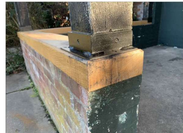
Image after to works showing new timber plates
