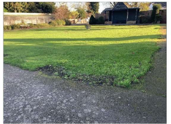
Ground surface following demolition of wall
