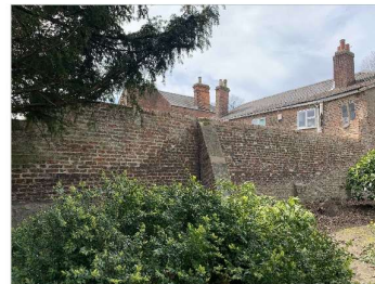
View of wall from N after partial collapse and rebuild
