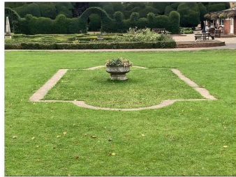
View from east after demolition.
