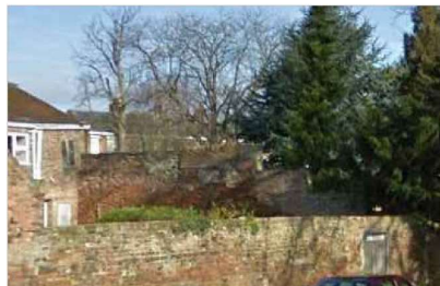
View of wall from SE prior to partial collapse and rebuild
