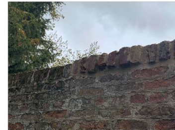
Detailed view showing capping course set in lime mortar
