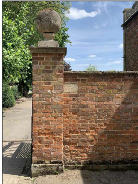
South pillar - top section rebuilt
