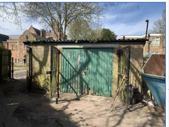
View of gardener's store door to be replaced
