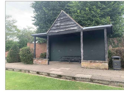
Image of shelter prior to works
