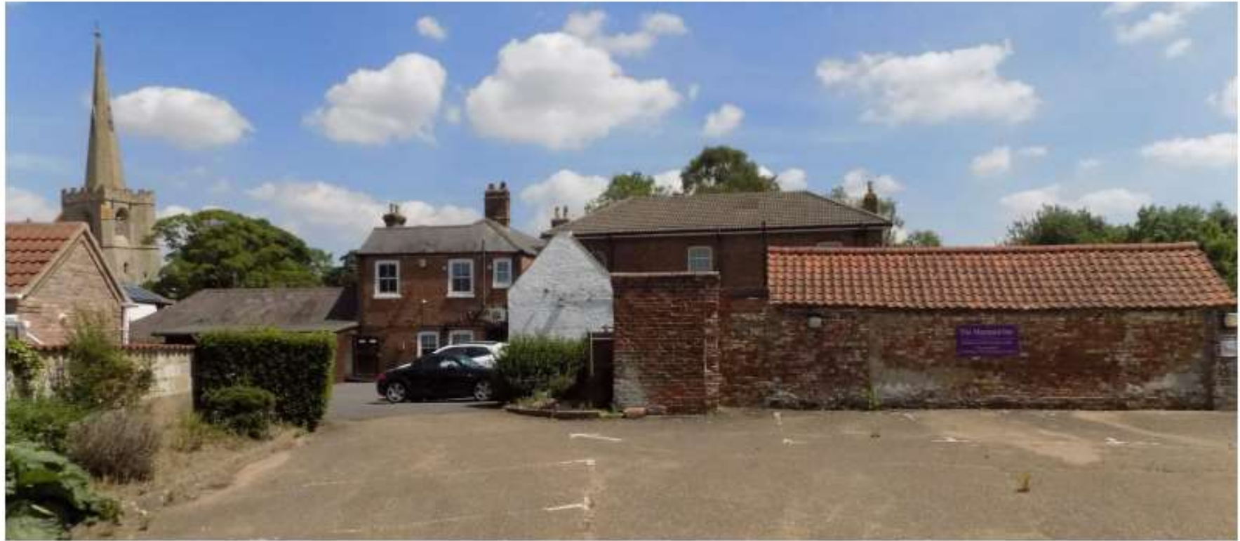
P5 – west elevations seen from beyond the garage.
