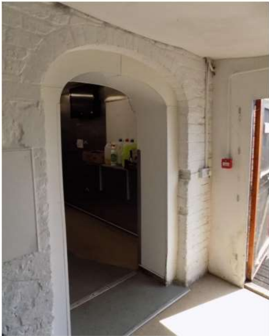
P17 – double elliptical arch to former stable.
