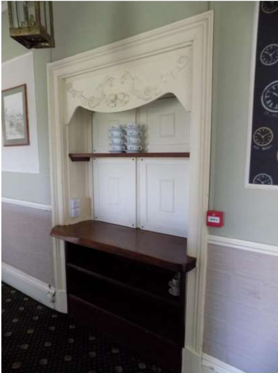
P28 – original door architrave and lining to front door.
