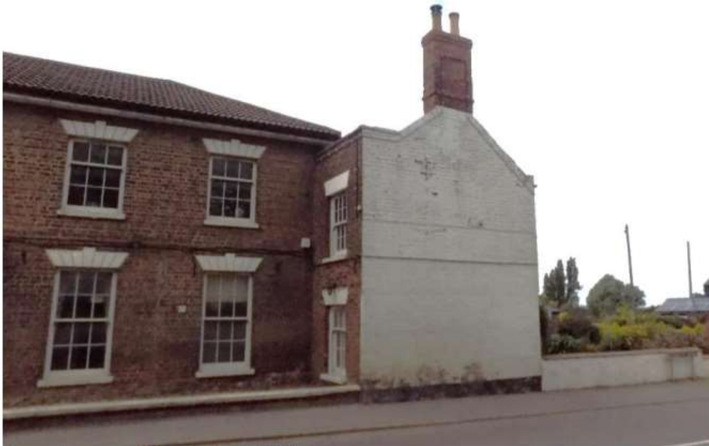
P7 – east elevation. note the parapet front to building 2.
