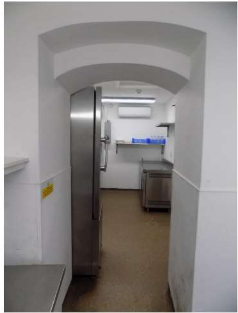
P18 – altered, reduced, and plastered double elliptical arch to stable.
