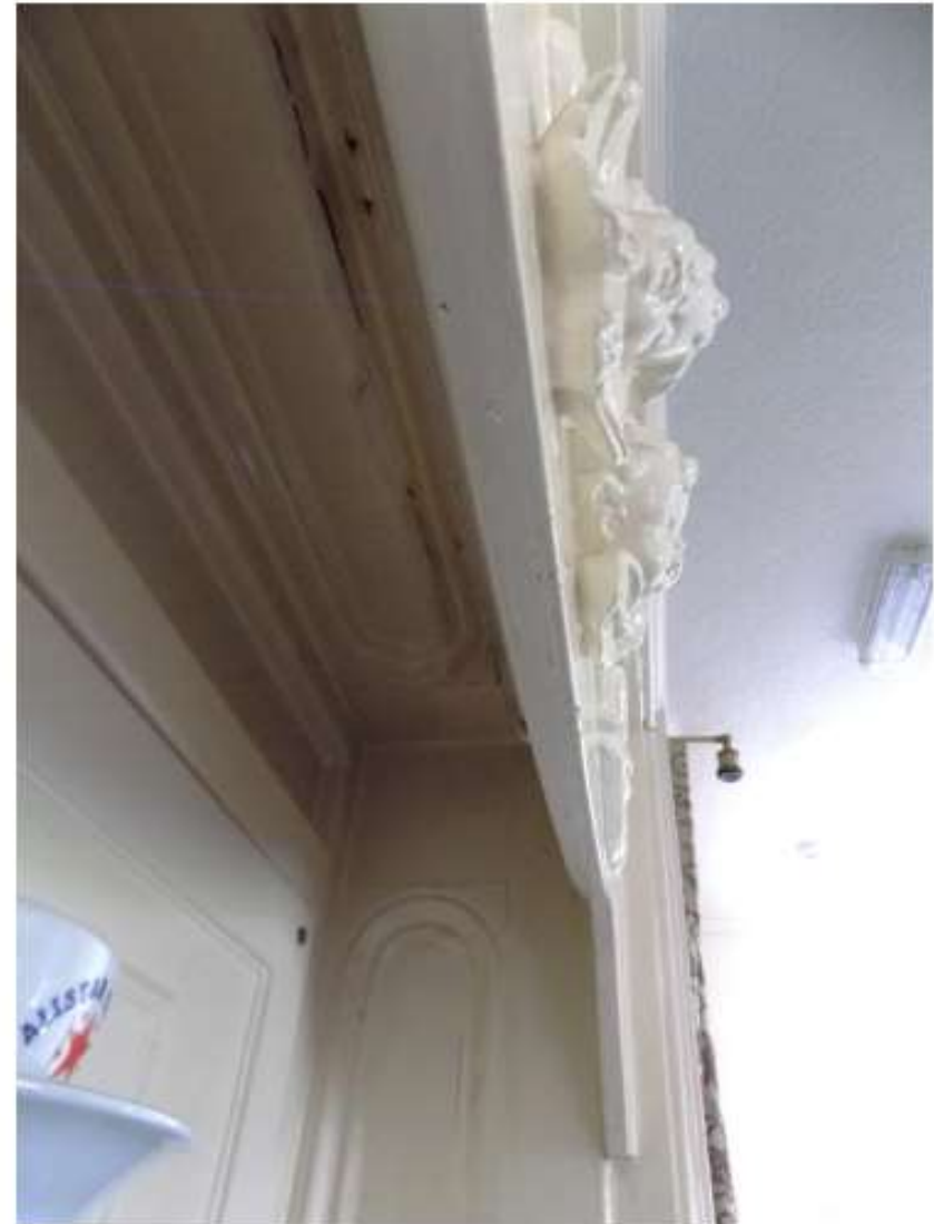
P28 – original door architrave and lining to front door.
