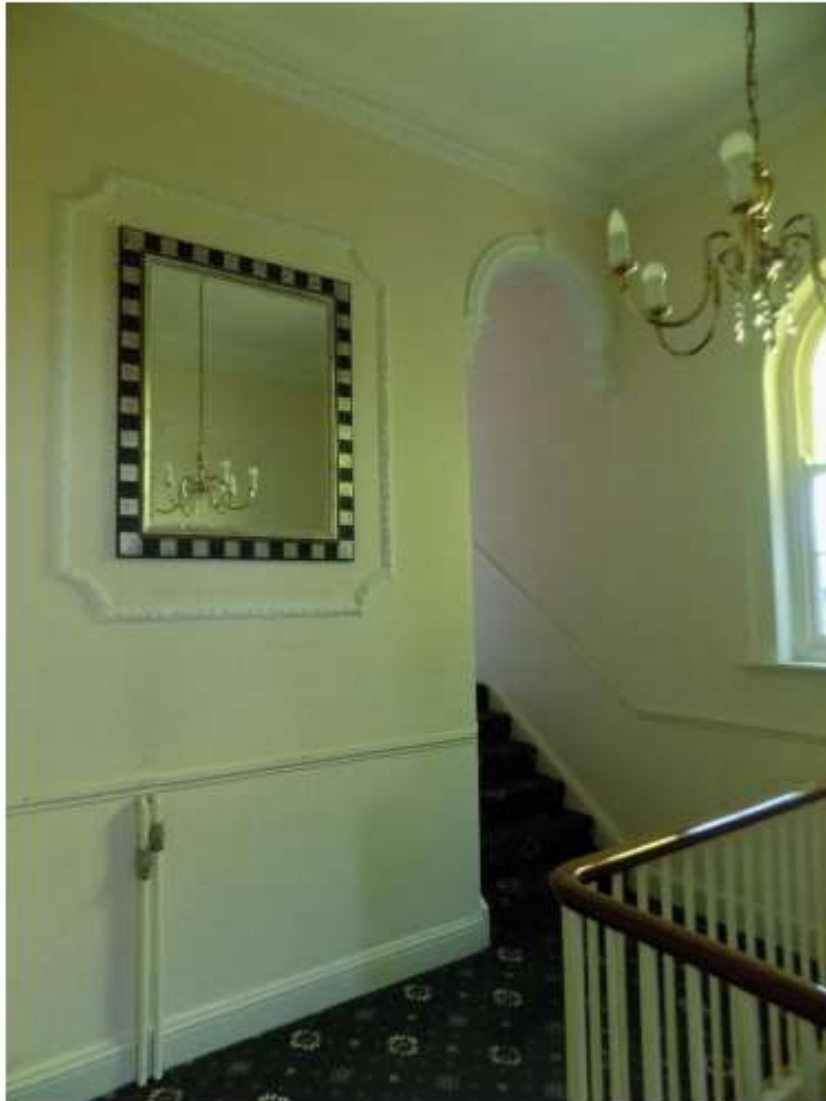
P23- steps to passage from the staircase hall to rooms FF1, FF2 and FF3.
