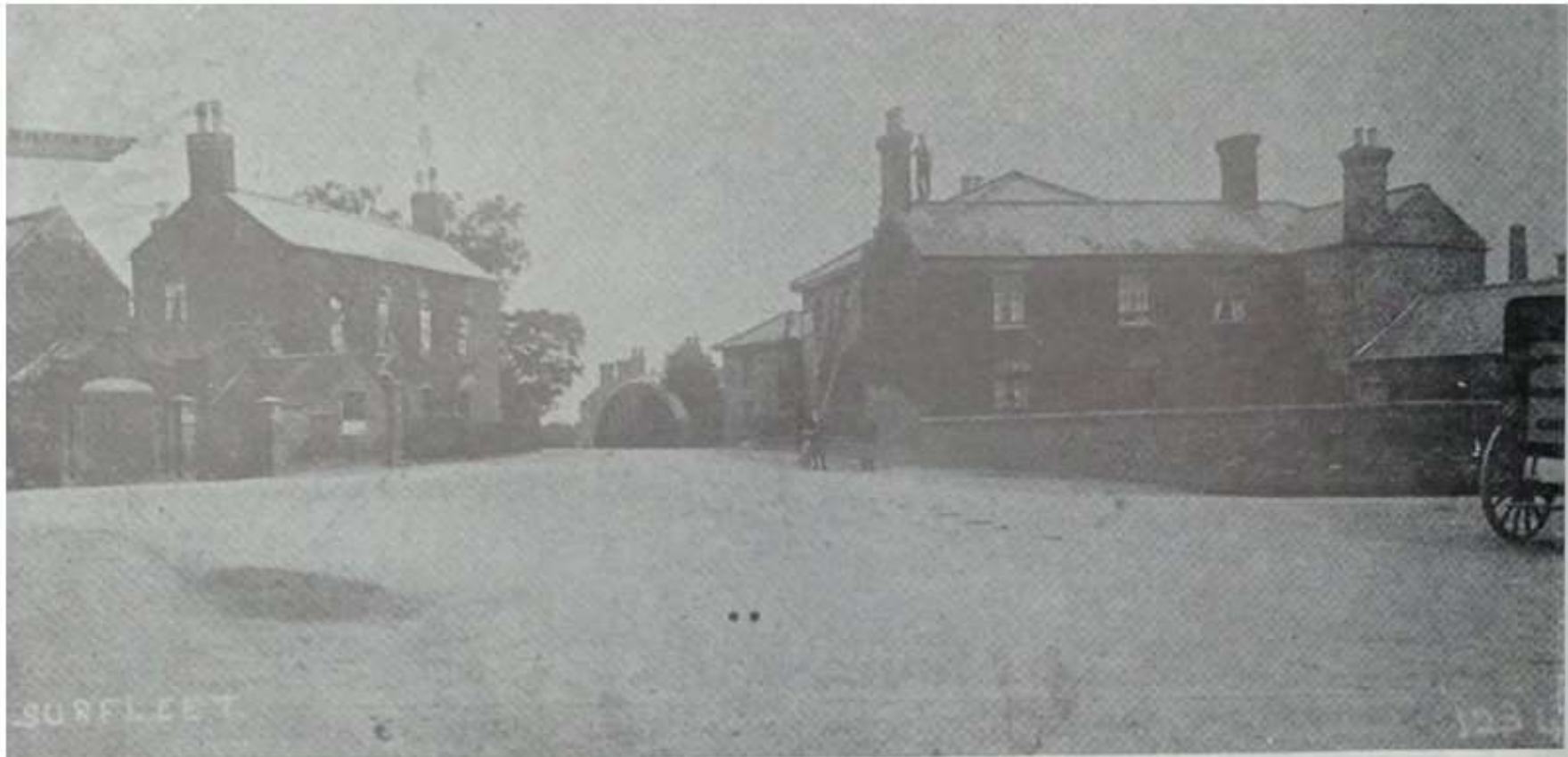
Above: Mr. Flowers, Surfleet bricklayer repairing chimney of Ivy house (now part of the Mermaid Inn).
