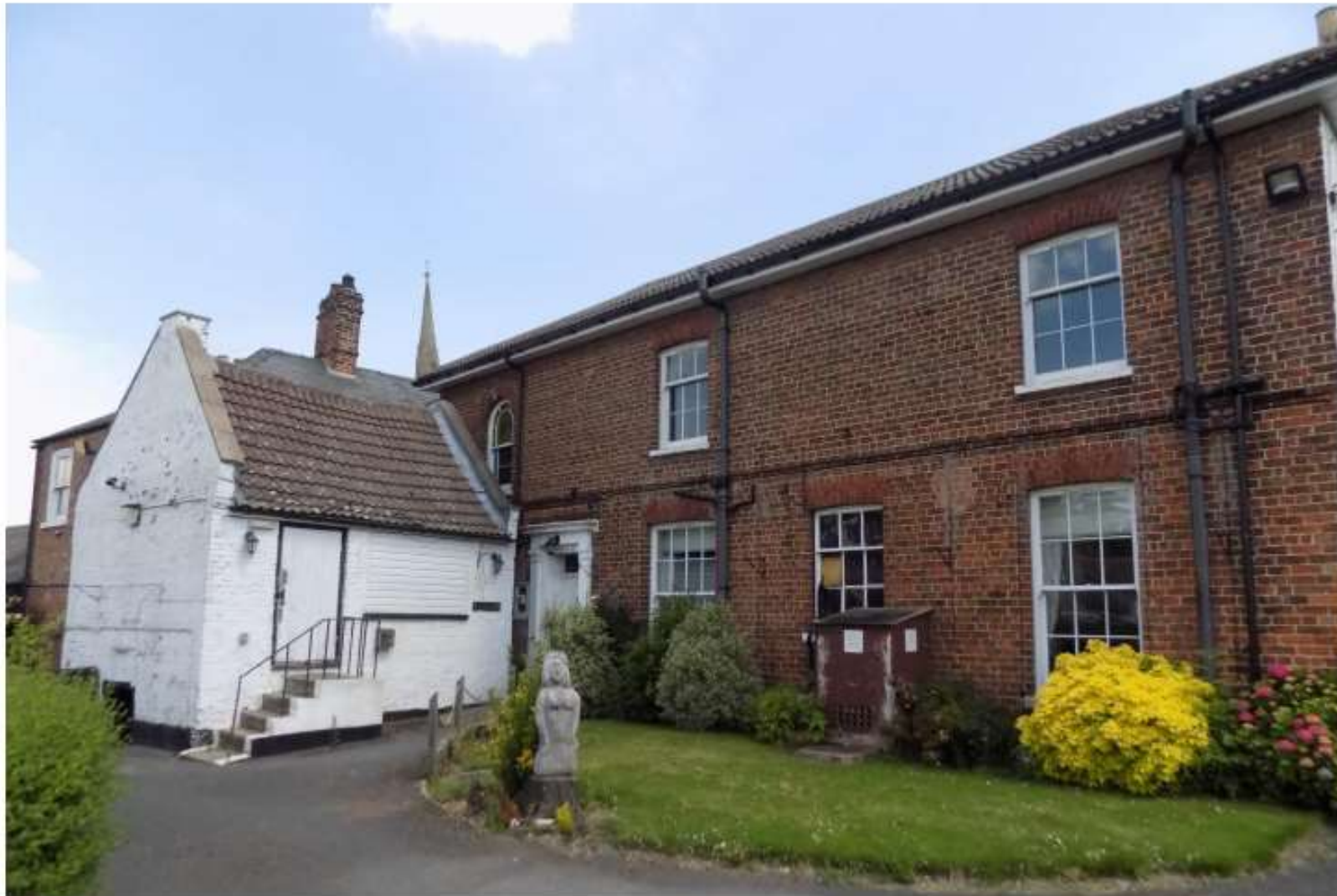
P6 – west elevation, building 1 is the earliest surviving building on this site and once detached.
