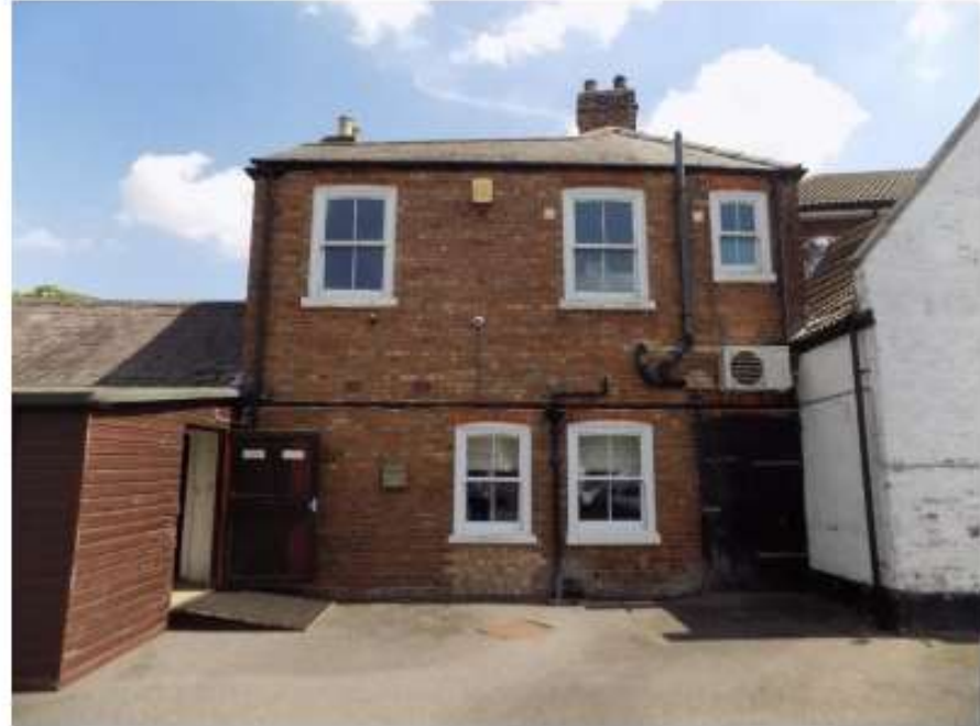
P8 – west elevation of building 5.
