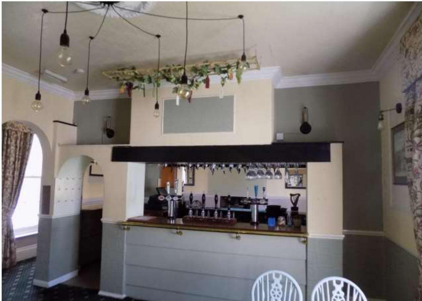
P25 – GF1, principal room of Building 4 contains an original cornice. Structural supports on walls to either side of the bar hold up what remains of the original chimney breast.
