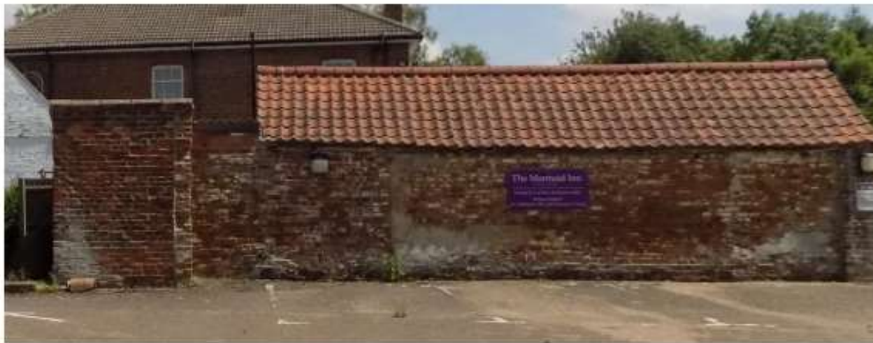
P13 – west elevation of garage and W.C.
