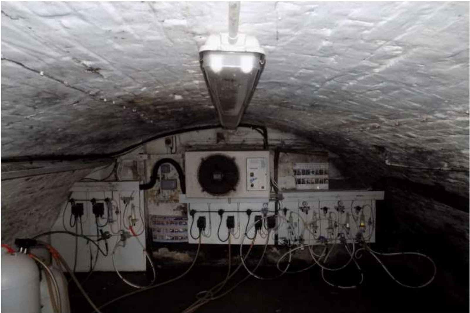
P16 – barrel vault to Building 1.
