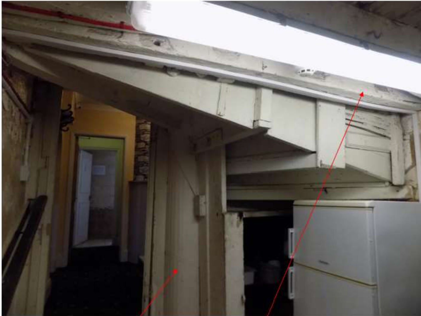
P24 – below the stairs, note the central column and some reused timbers.
