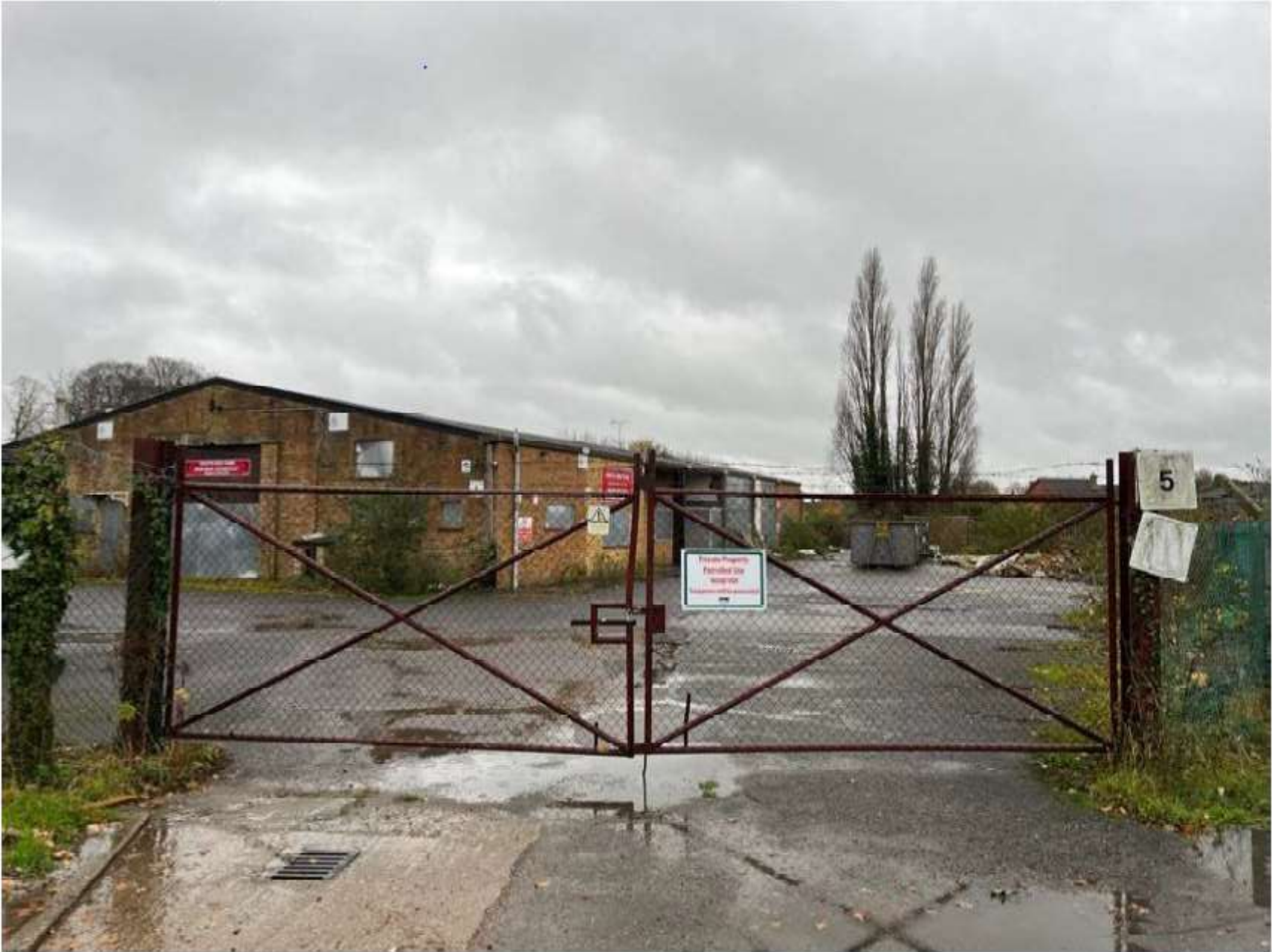
Former boxing club central in site
