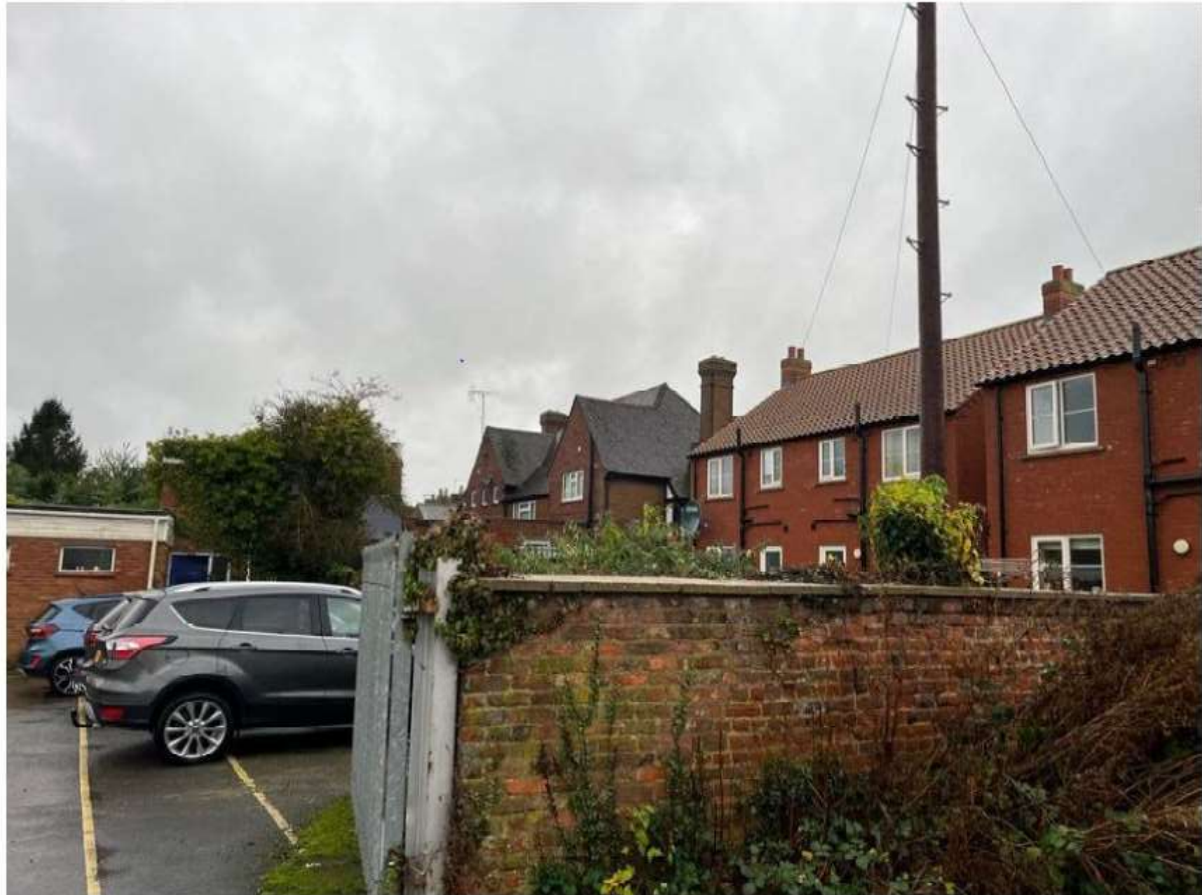
Rear of properties 74-76 fleet street
