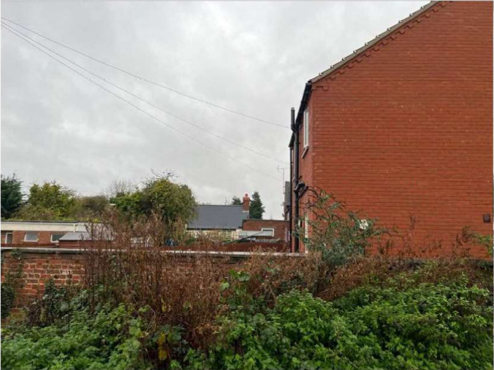
Gable end of 76 fleet street
