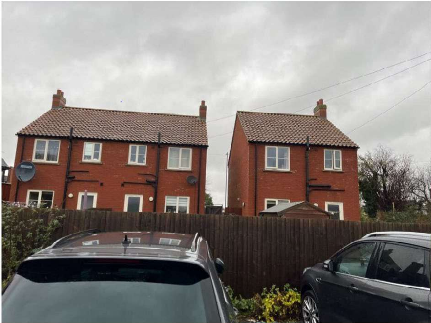
Rear of 74 – 76 fleet street
