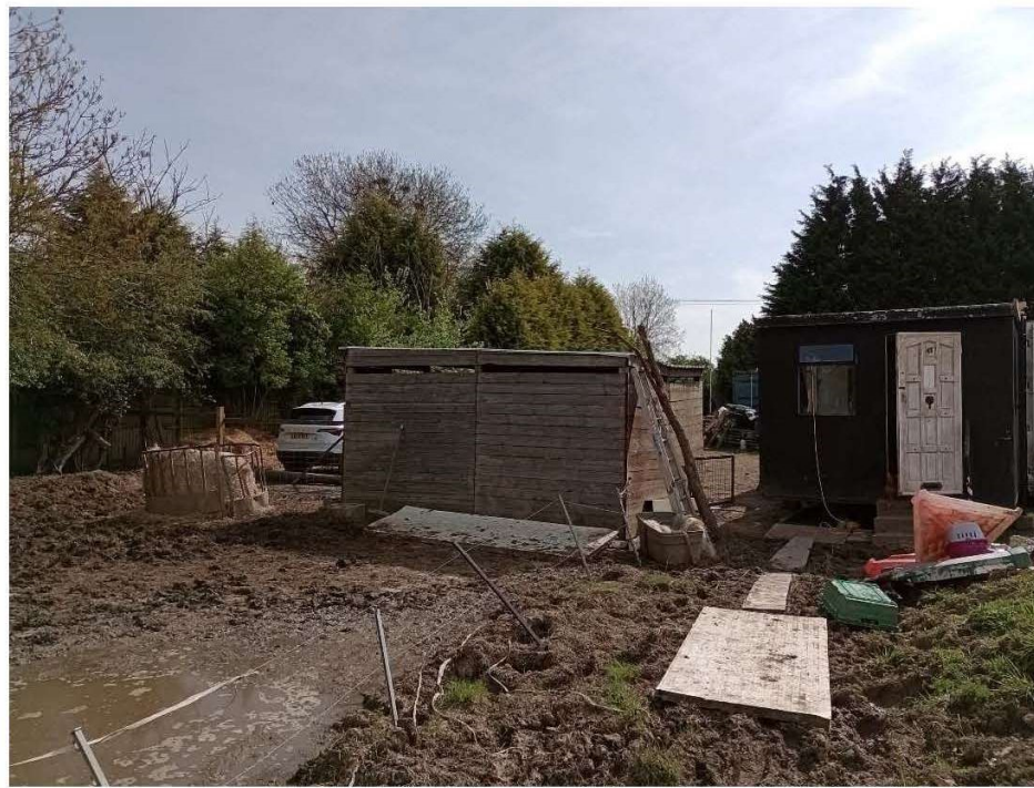
Existing buildings on site looking towards access.
