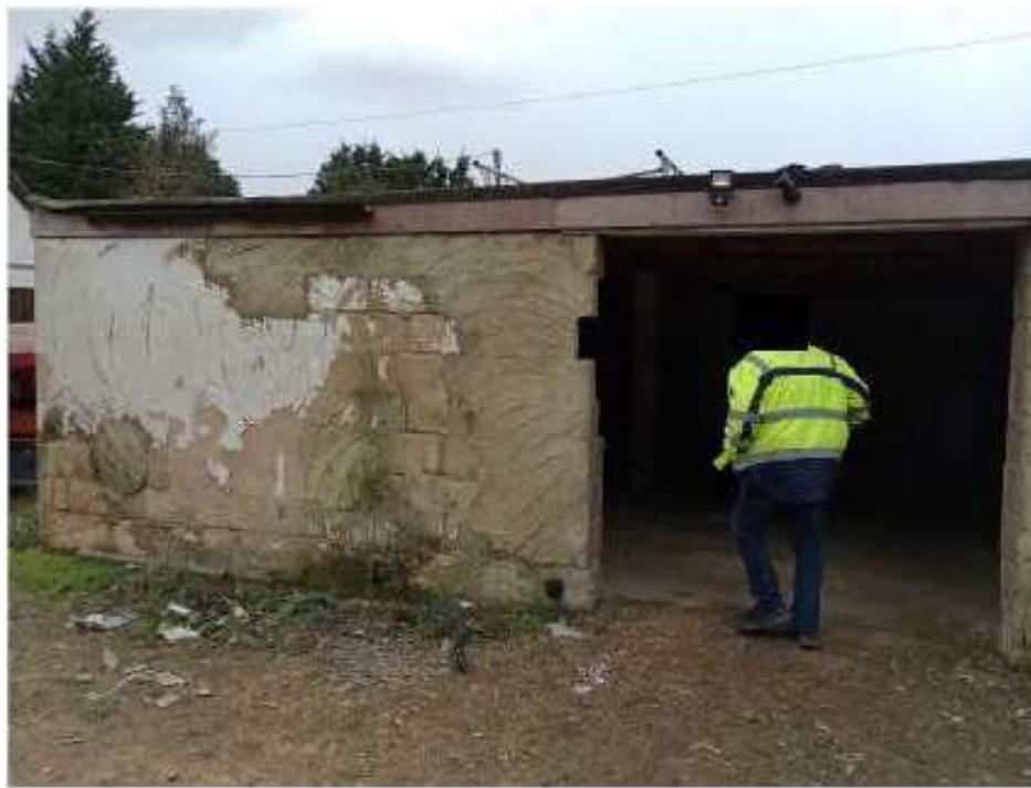
Photo of rear of stable
