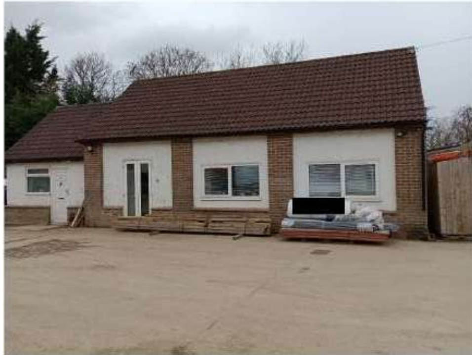
Photo of Office/quasi residential to be turned back into a garage.
