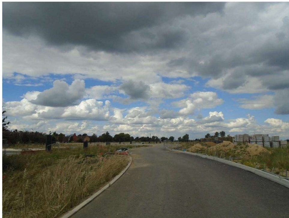
Present internal roadway
