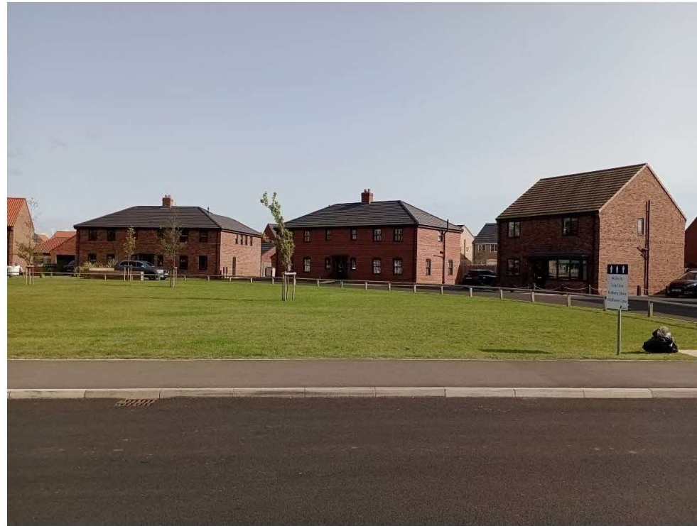
Views of the front of Holbeach Meadows (Part of first houses constructed)
