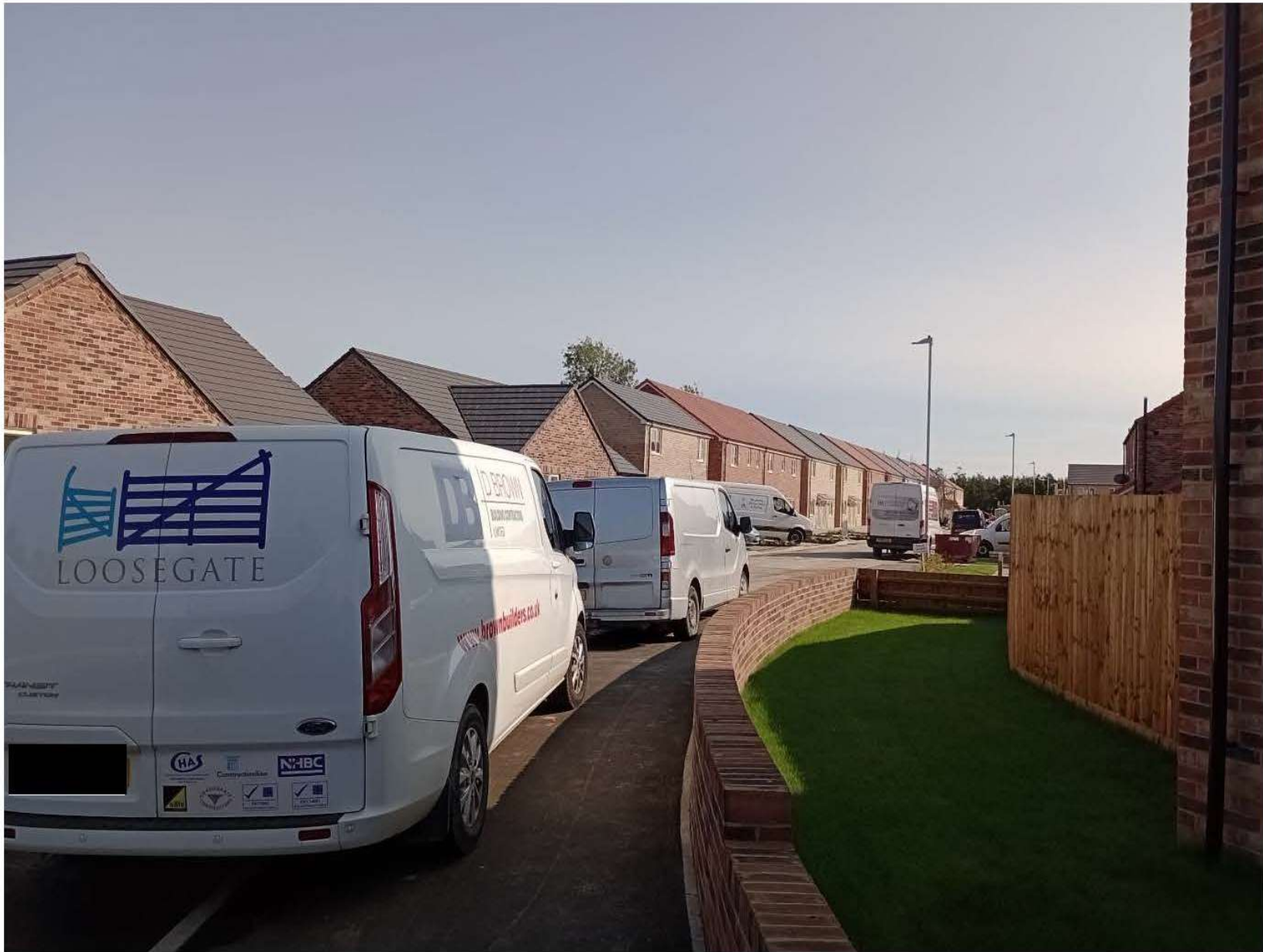
View of affordable housing on main site already constructed
