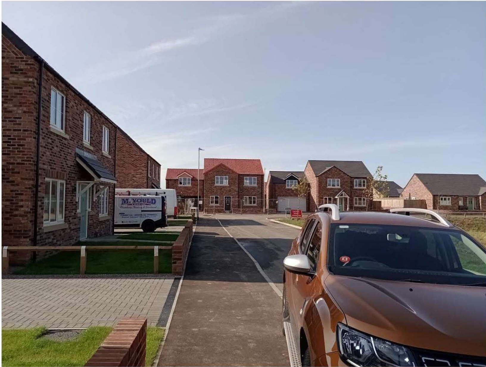
Dwellings constructed on main site
