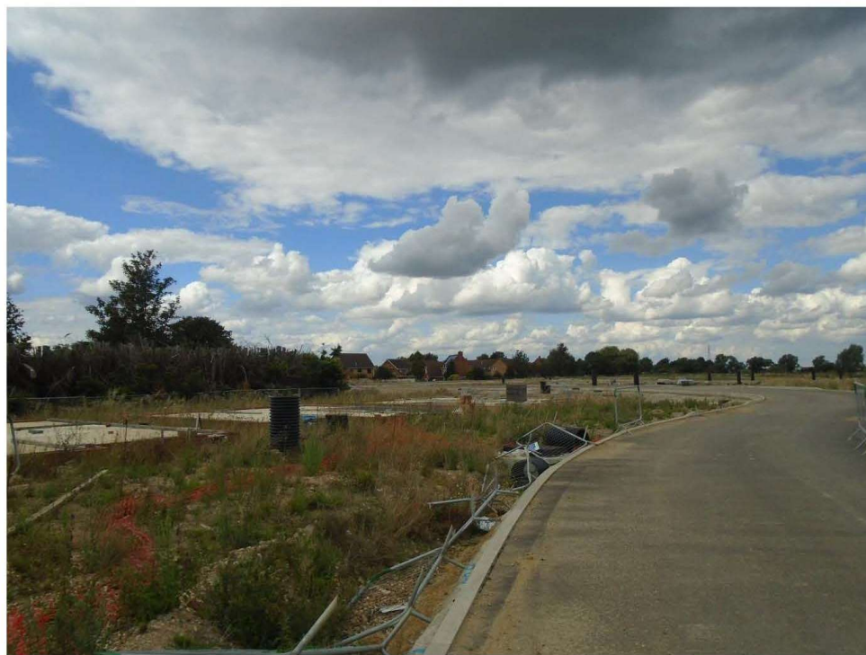
Plots near entrance under construction
