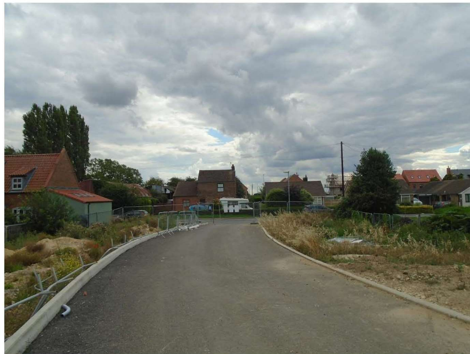
Entrance roadway facing Roman Road
