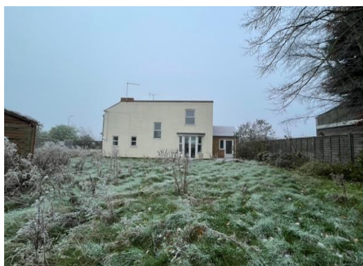
Photograph 2: Eastern elevation of the dwelling and the garden
