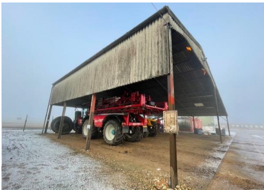
Photograph 10: View of Building 3
