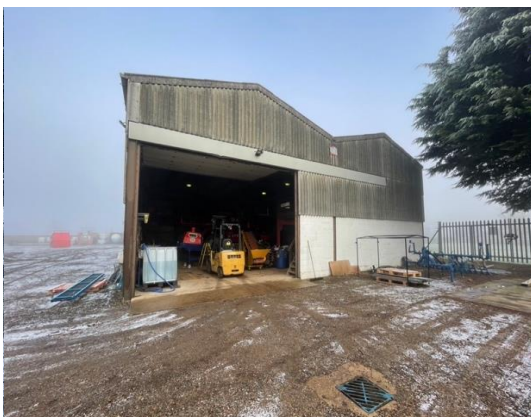
Photograph 14: Southern elevation of Building 5
