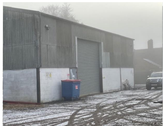
Photograph 15: Western elevation of Building 5
