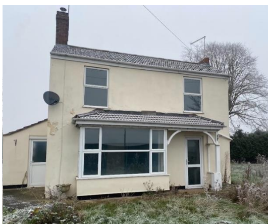
Photograph 4: Southern elevation of the dwelling
