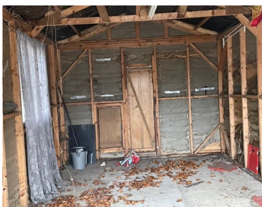
Photograph 6: Internal view of the timber garage
