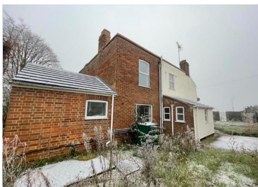
Photograph 1: Western elevation of the dwelling
