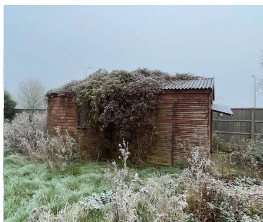
Photograph 5: The timber garage
