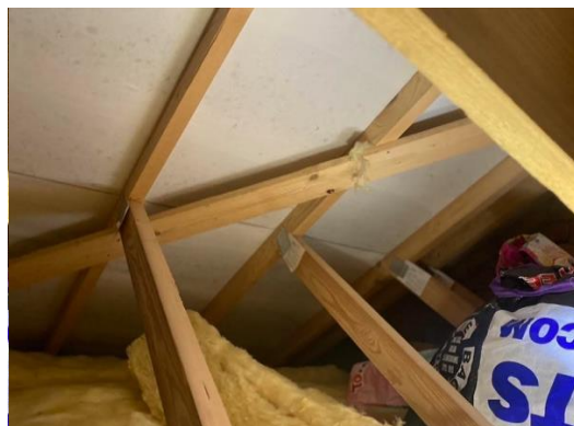
Photograph 3: Roof void within the northern extension
