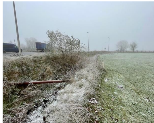
Photograph 32: North-eastern boundary ditch along the A17
