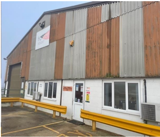
Photograph 8: Southern elevation of Building 2
