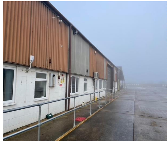
Photograph 9: Eastern elevation of Building 2
