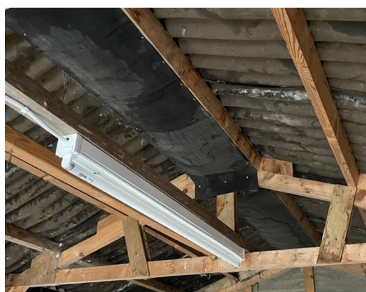
Photograph 7: Roof structure of the garage
