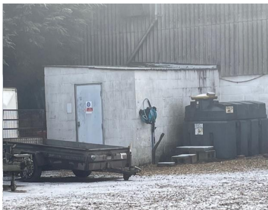
Photograph 16: Small concrete block room off northern elevation
