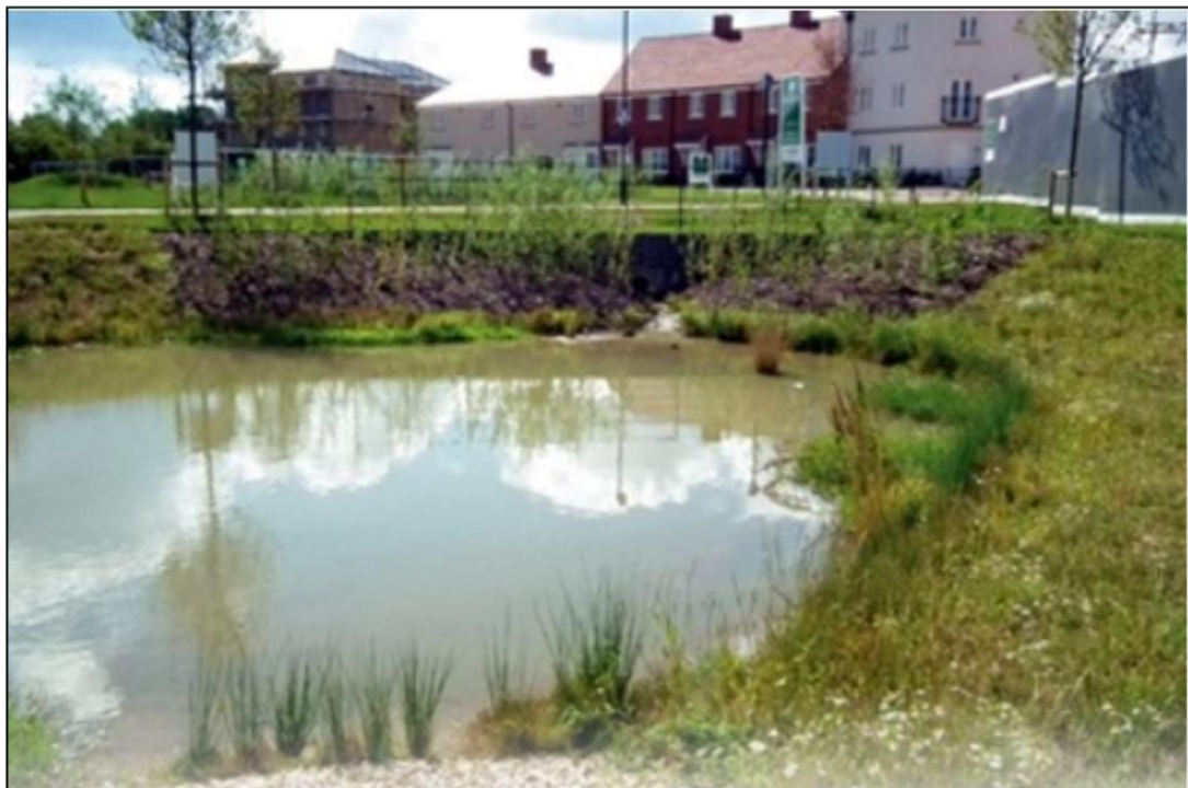
Figure 4-1: Example of Open Attenuation Pond with Planted Edges and Permanent Water
