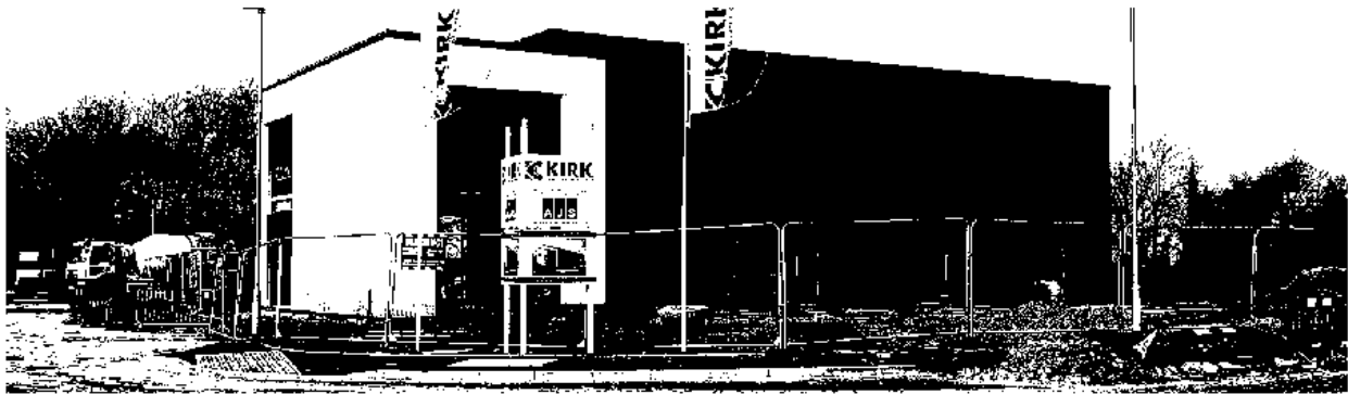
Figure 2: Unit currently under construction
