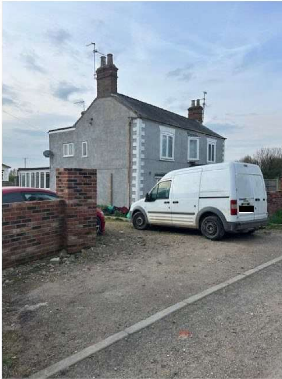
Above: No 184 Seagate & domestic access
