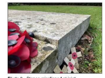
Photo 9 - Stones misaligned at joint
