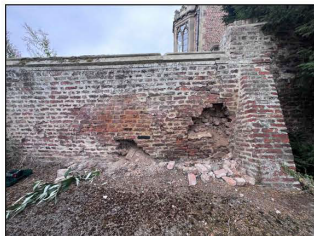
General view South elevation of wall
