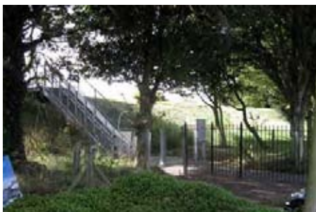
The water taxi stop connections with Springfields should be made more prominent
