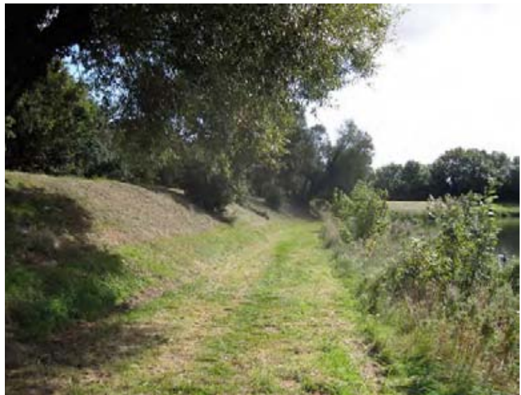
Spectators can use the flood banks to view waterspace events
