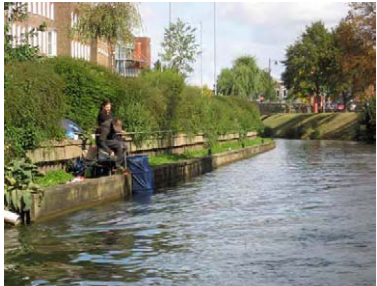
The existing moorings to the south of High Bridge and Taku Footbridge will need to be refurbished, extended and additional accesses created.
