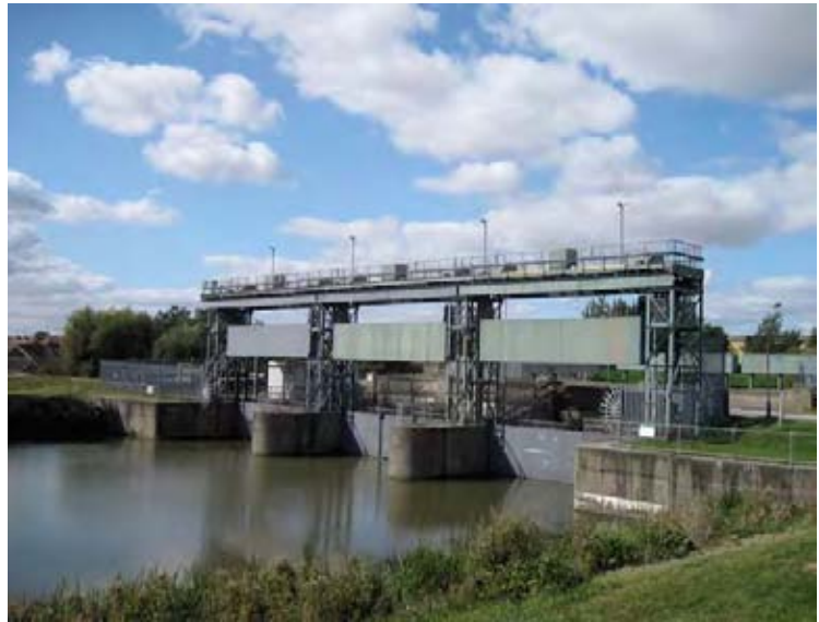
Marsh Road Sluice should be relocated downstream of the new non-tidal connection with the Vernatt's Drain. This will allow navigation between the River Welland and the Coronation Channel
