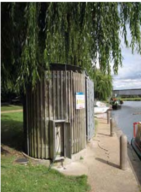
Example of a discreet small scale waterway facilities block, Great River Ouse, Ely
