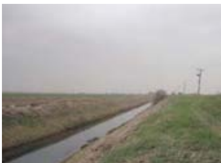
The Black Sluice Navigation north of the A151
