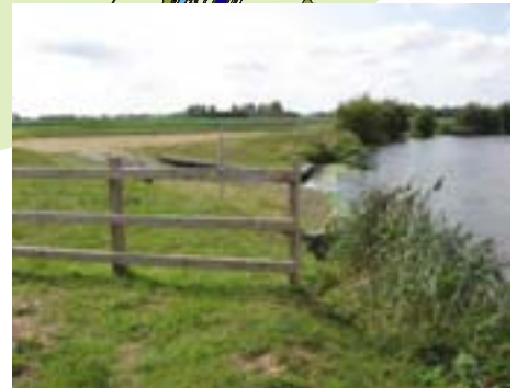
Macmillan Way deviates around Surfleet slipway
