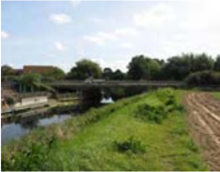
A16 Bypass road bridge
