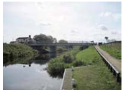
Bars Bridge carries the A151 over the River Glen, Pinchbeck West
