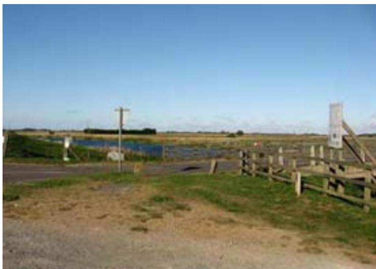
Fencing and signage detract at Crowland Bridge
