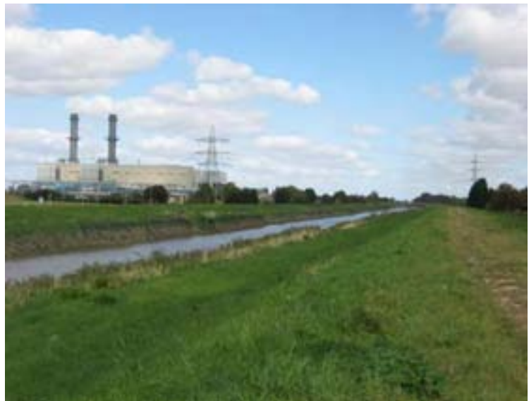
Spalding Power Station and pylons dominate the view
