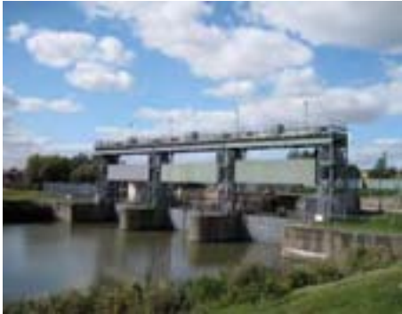
Marsh Road Sluice
