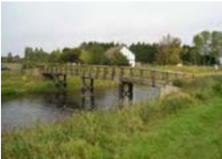
Jobson's Bridge, Vernatt's Drain
