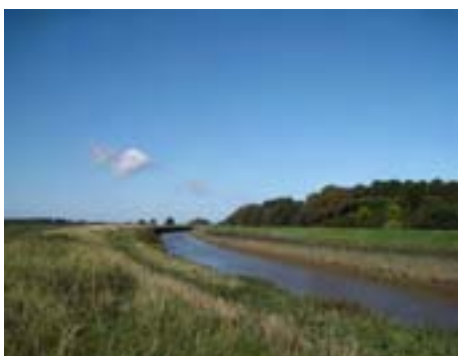
The Tidal River Welland constrained by flood banks
