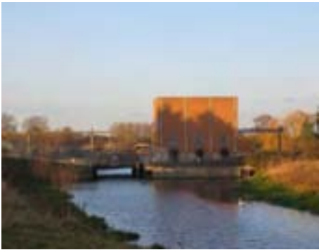
Peakirk Pumping Station, The Folly River
