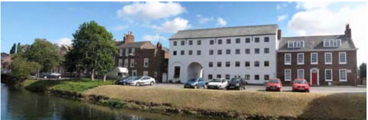
Merchant houses and the warehouses have lost their connectivity to the river
