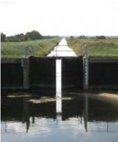
The Delph Drain looking west
