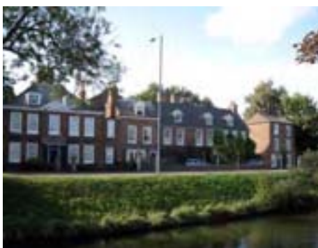
There are many fine Georgian buildings set back from the river
