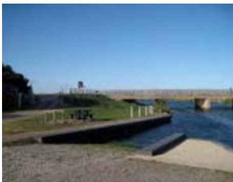
Crowland Slipway and Bridge
