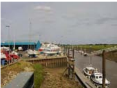
Fosdyke Yacht Haven, Fosdyke Bridge
