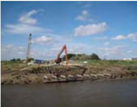
'Fosdyke slipway with new careening berth under construction , Fosdyke Bridge
