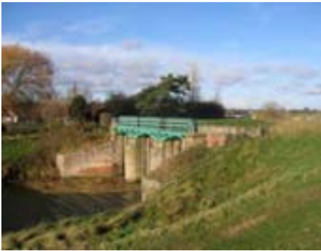
Vernatt's Drain Sluice
