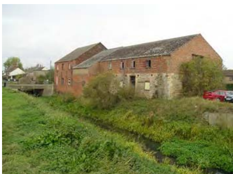
Old warehouses line the waterway, Bourne
