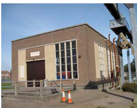
Pode Hole Pumping Station
