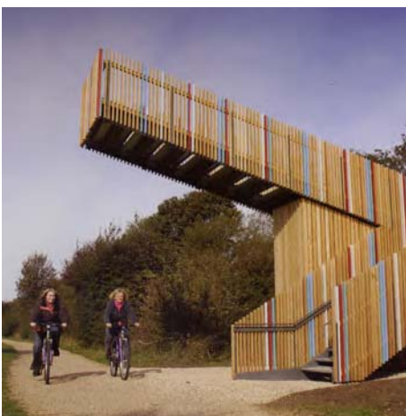
The Boston Pendulum on the Water Rail Way creates a destination point along the route (Ref: Our Vision for the Lincolnshire Waterways, LWP, 2008)
