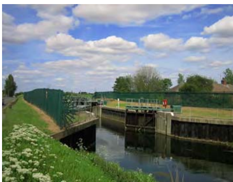
Fulney Lock, River Welland, Spalding
