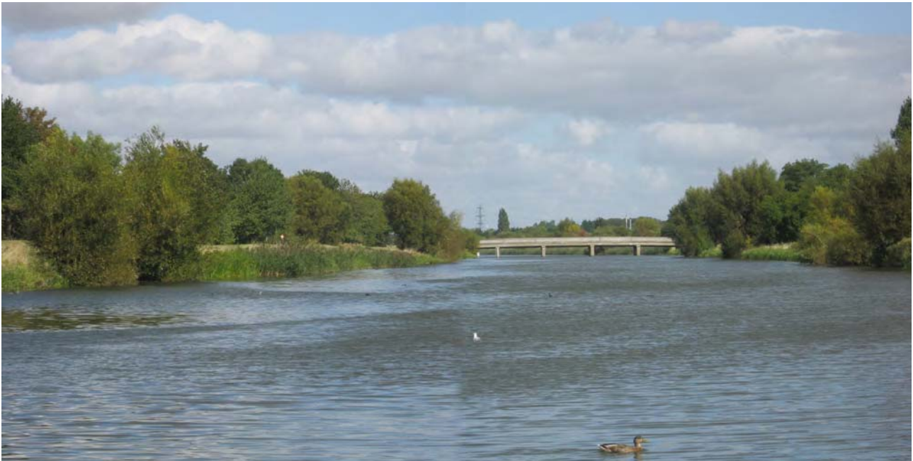
The broad waterway of the Coronation Channel around Spalding's eastern boundary
