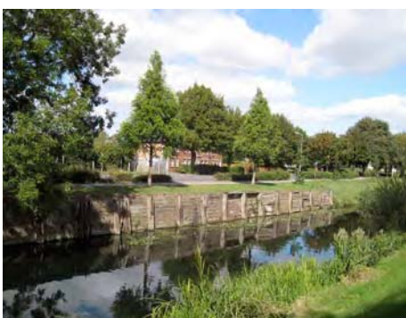
The Gasworks Wharf, Spalding
