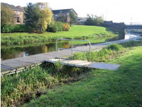
Standing moorings off the bank maintains marginal vegetation and helps improve security
