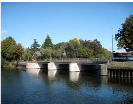
The low 'air draught' of Cowbit Road Sluice will be to be addressed to allow larger craft to navigate on the Coronation Channel
