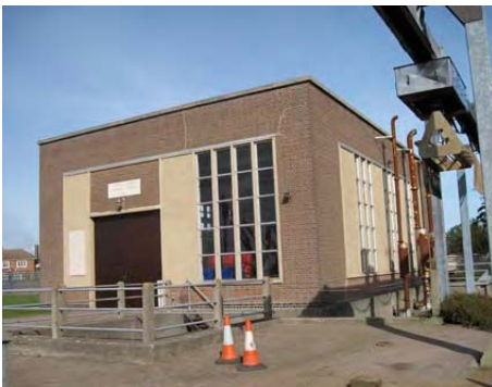
Pode Hole Pumping Station
