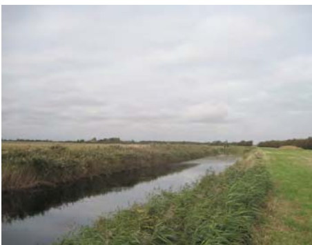
South Drove Drain
