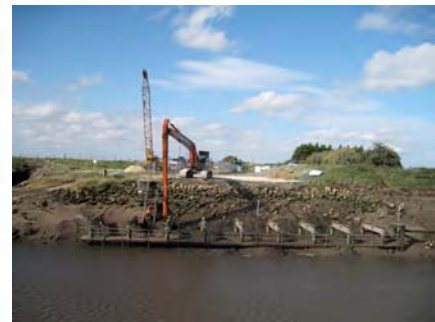
Careening berth, upstream of Fosdyke Bridge
