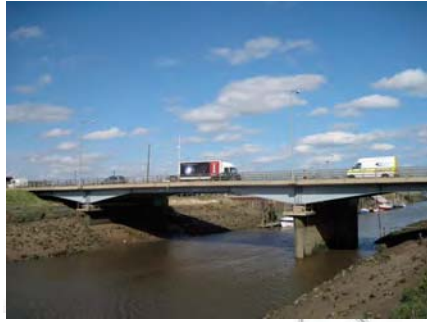
Fosdyke Bridge, River Welland
