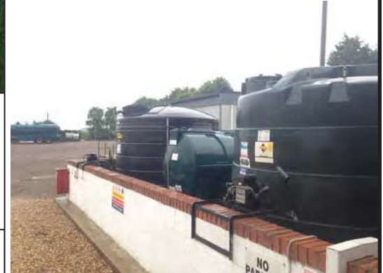
PH06: Bunded aboveground fuel tanks.
